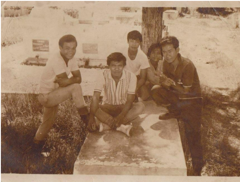
Figure 12. Early Cemetery Workers resting on the Circle section: From left to right: Danilo Babli-ing, "Pidring", and an unidentified worker, "Amping", and Benjamin R. Dizon, the City Cemetery Caretaker, ca. 1960s. Dizon Family Photo Collection
