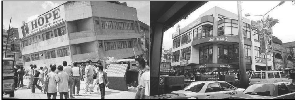
Figure 4. The Royal Inn at the corner of Lapu-Lapu and Rajah Soliman Streets was damaged in the 1990 earthquake. In its place is Jollibee Magsaysay.
